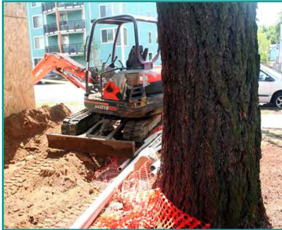
Tree on property line during construction
