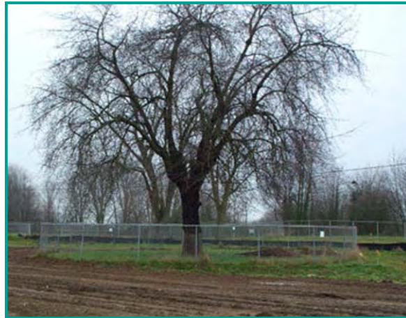
Tree protection fencing
