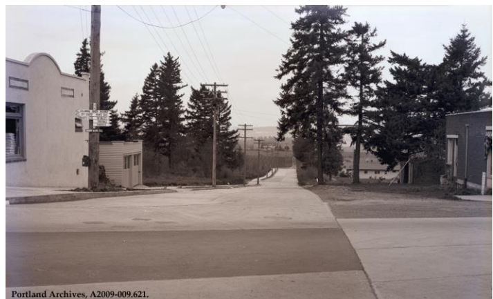
Same section of 82 nd from NE Sandy to NE Prescott after widening, City of Portland Archives, A2009-009.621
